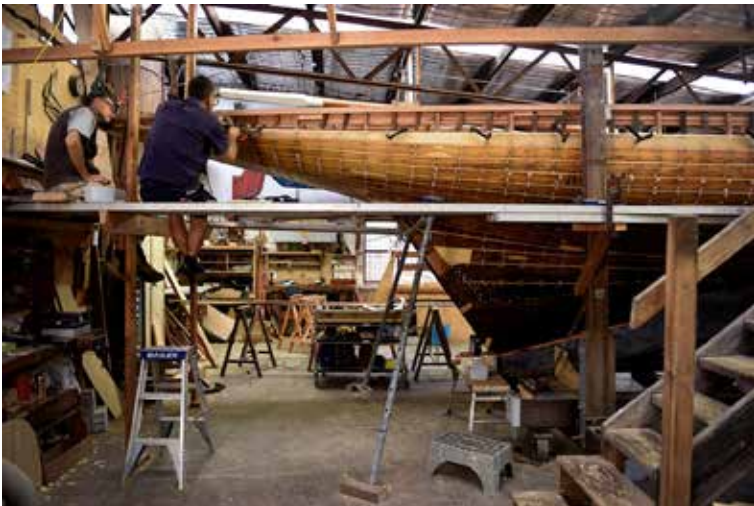
Dismantling and replanking. Images: Gerry Colley.
